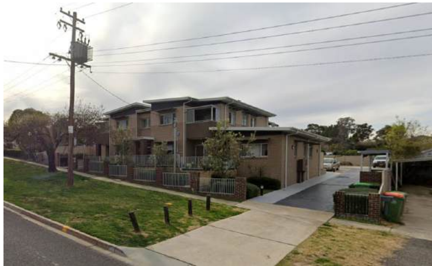
EXISTING 2 STOREY MULTI UNIT DEVELOPMENT
