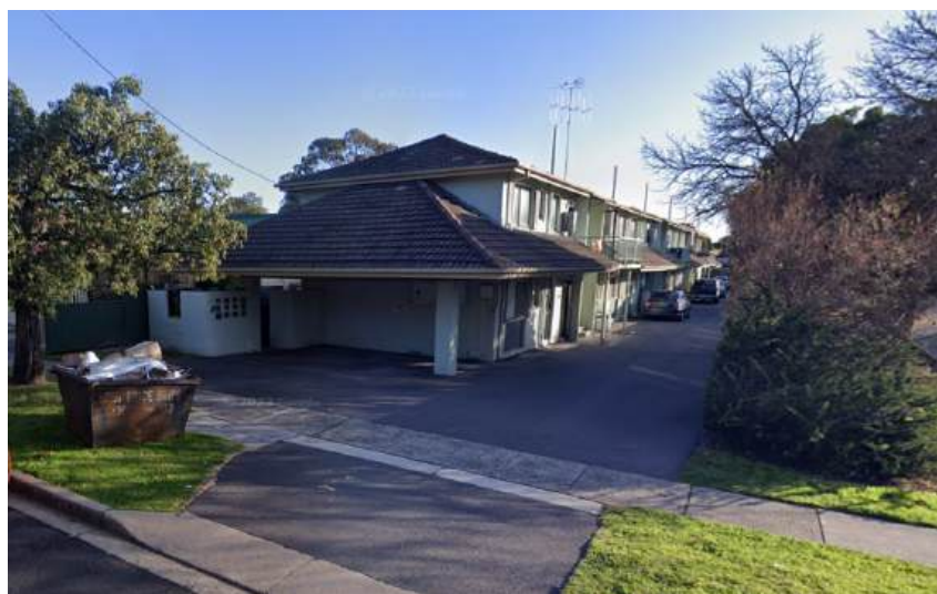
EXISTING 2 STOREY MULTI UNIT DEVELOPMENT
